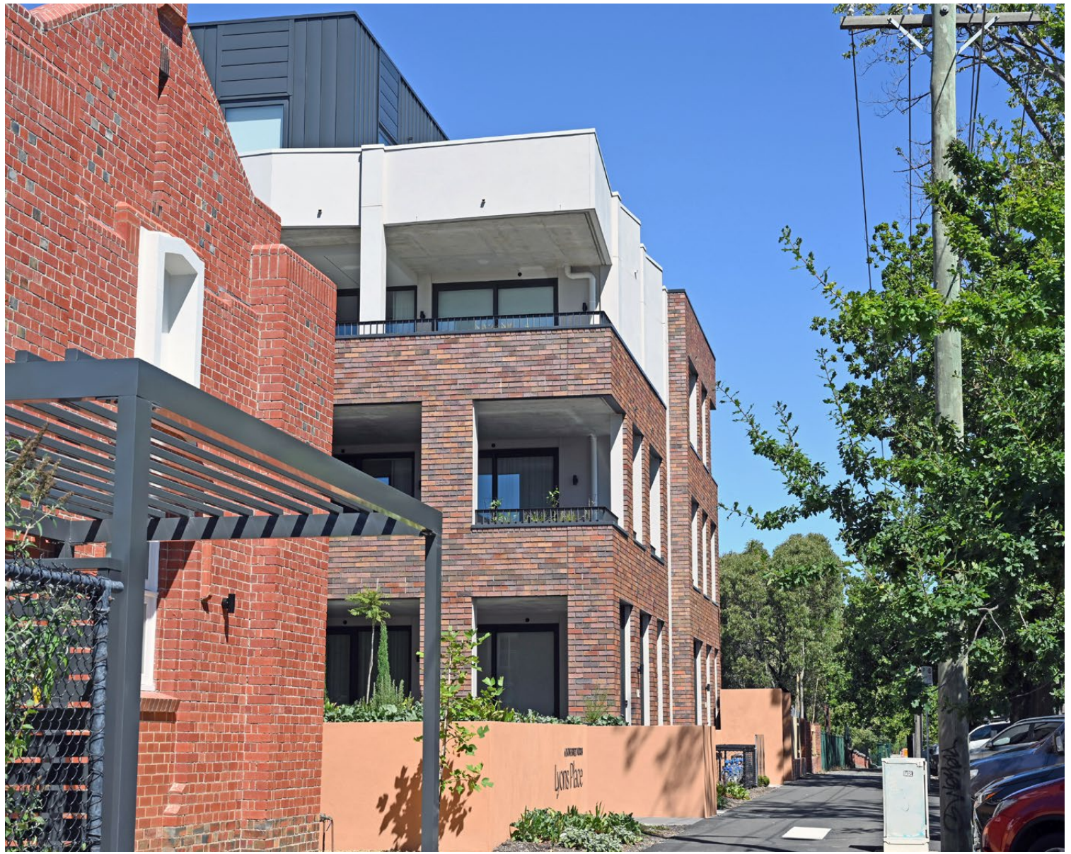
New higher-density development on Lyons Street North, demonstrating a three storey street wall/frontage with upper levels setbacks.
