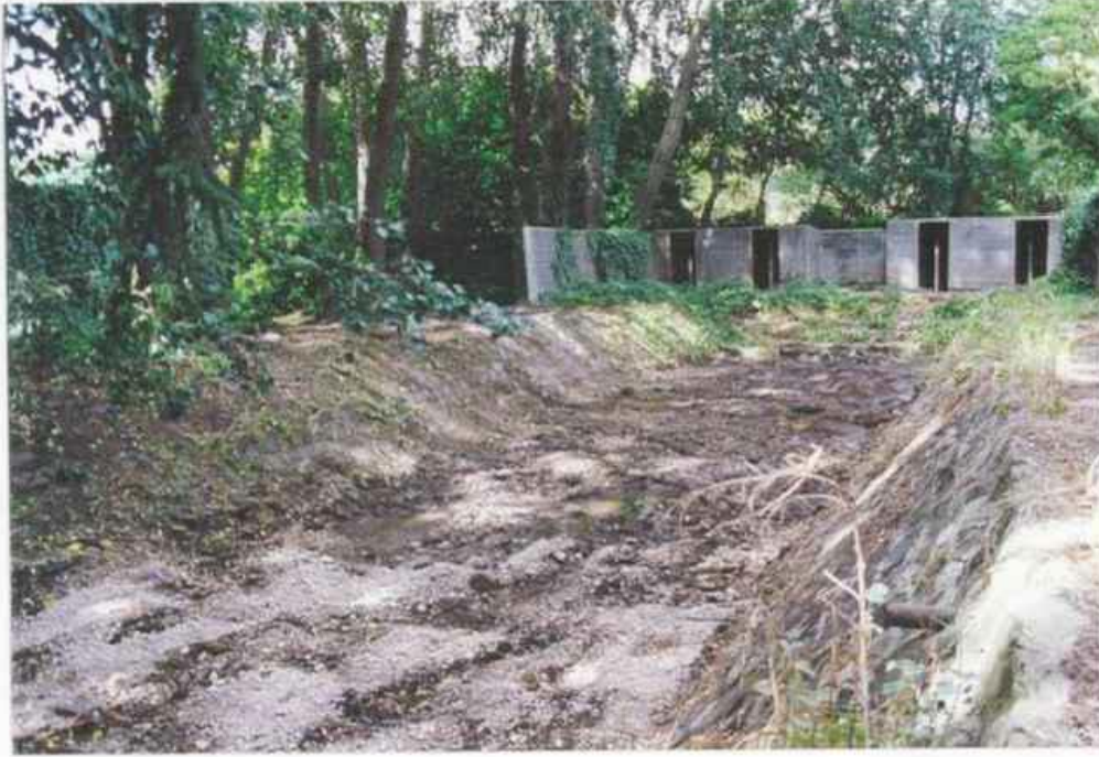
October 1993 Landscaping in progress.
