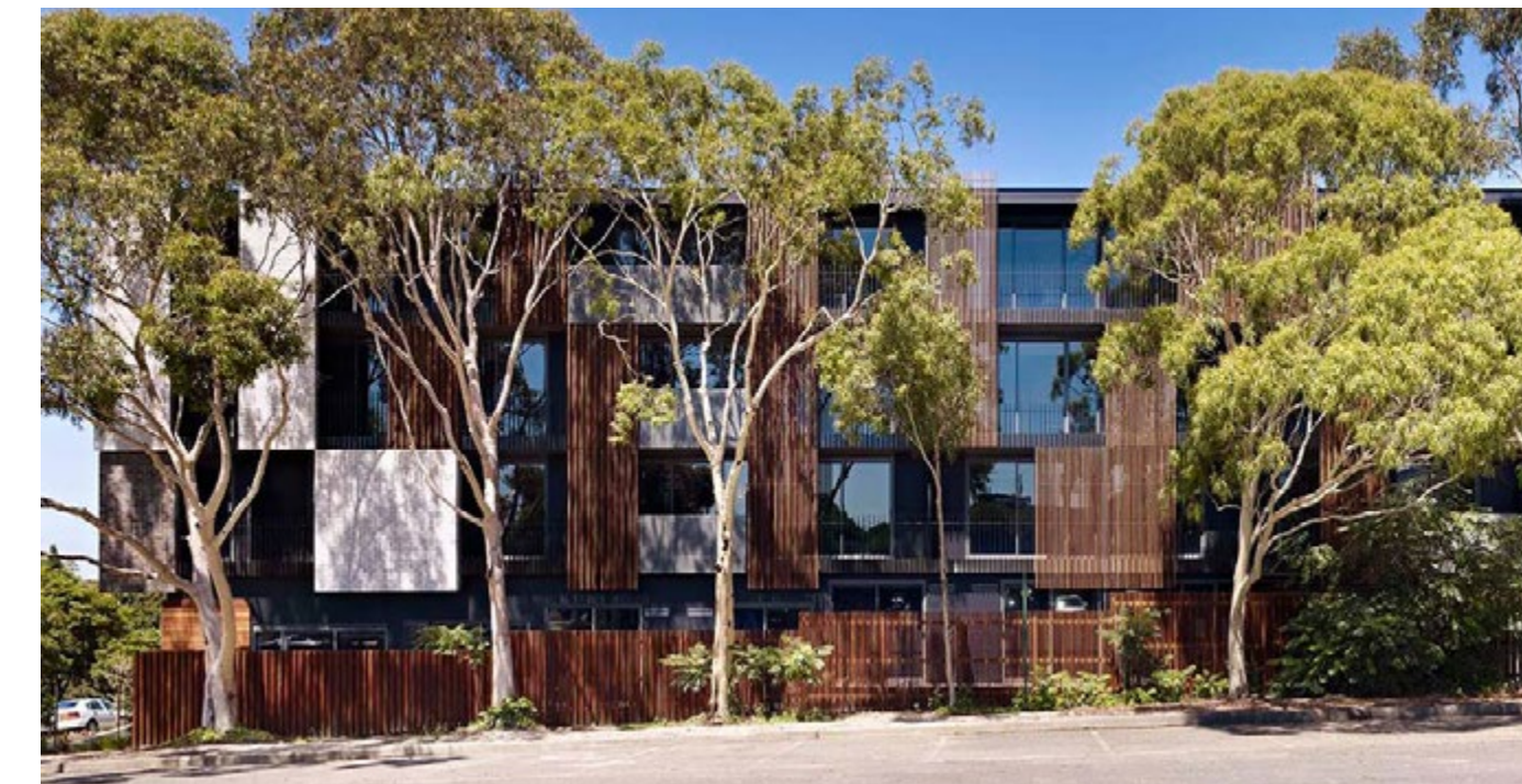
Figure 38: Medium-density housing - Box Hill VIC
