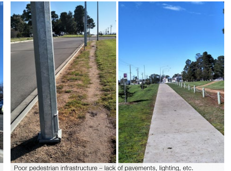
Poor pedestrian infrastructure – lack of pavements, lighting, etc.
