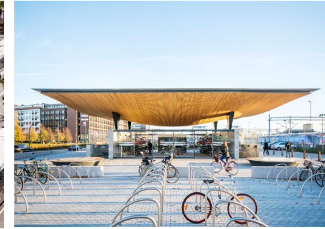
Figure 31: Pedestrian-friendly railway station - Helsingborg - Sweden
