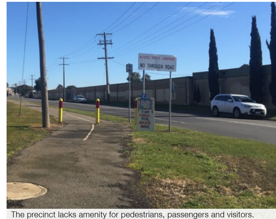
The precinct lacks amenity for pedestrians, passengers and visitors.
