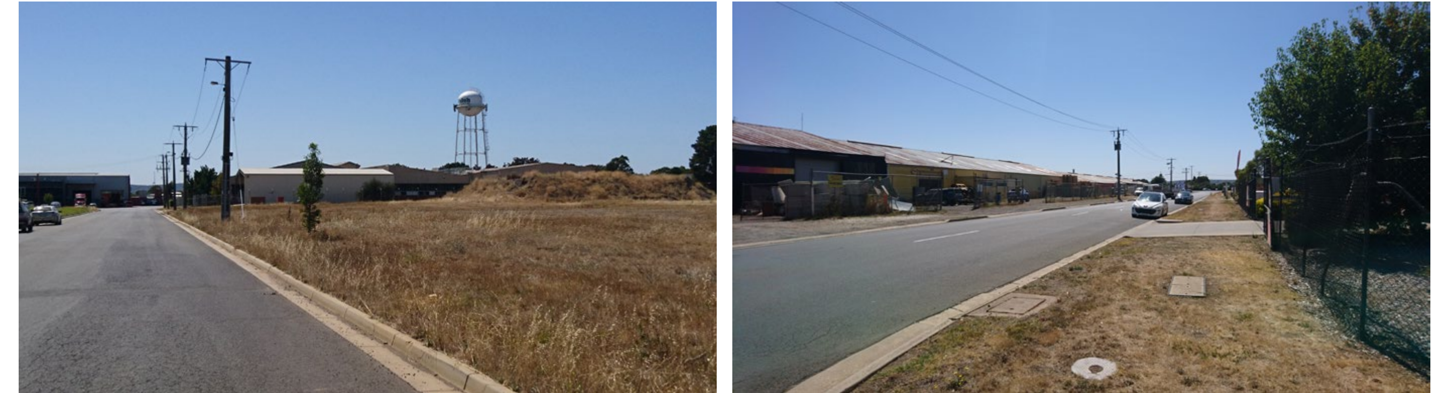
Figure 25: Existing Condition of Industrial Areas
