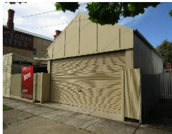
Figure 24. View of garage to the west. (Source: GML, October 2024)
