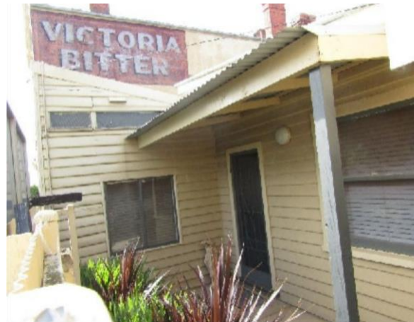
Figure 22. View of west extensions and outbuildings. (Source: GML, October 2024)
