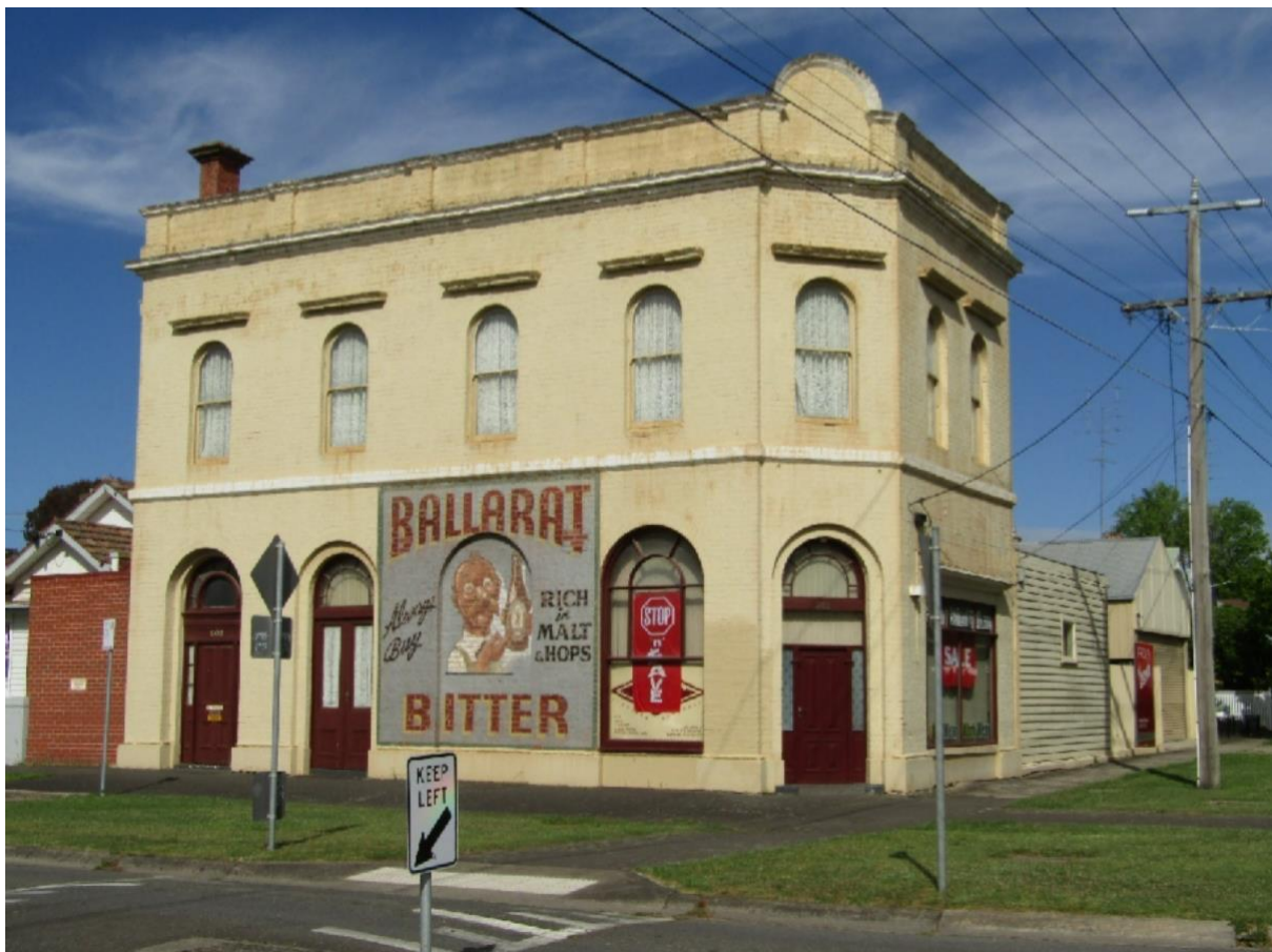
Figure 1 View of 202 Lyons Street South, looking west. (Source: GML, October 2024)
