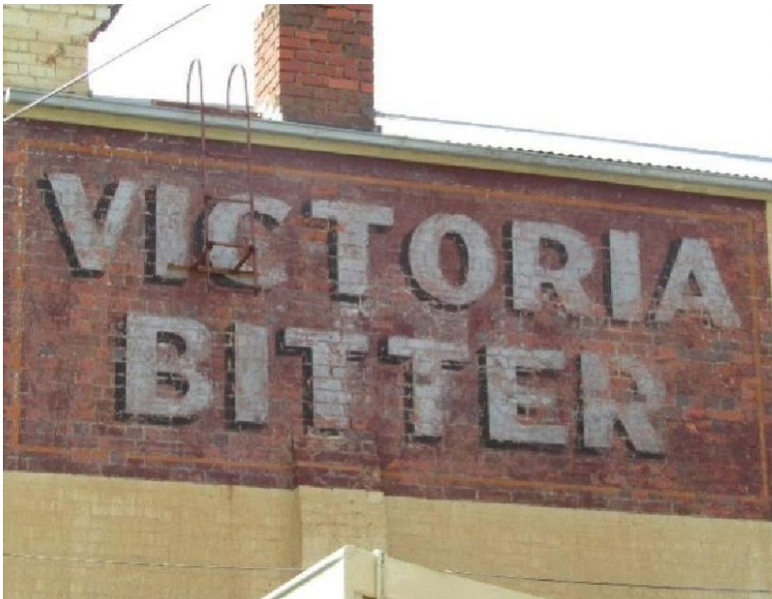
Figure 26. View of painted Victoria Bitter sign on west elevation. (Source: GML, October 2024)
