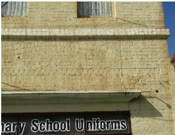
Figure 21. View of northern elevation facing Eyre Street, showing steel beam and brickwork arch. (Source: GML, October 2024)
