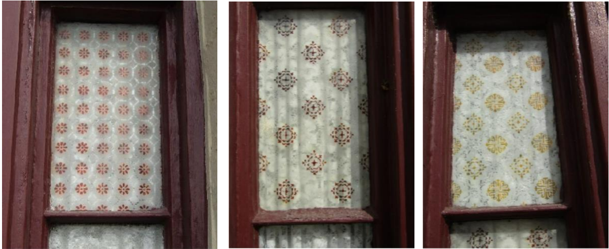
Figure 20. Decoration to glazed sidelights on east elevation. (Source: GML, October 2024)
