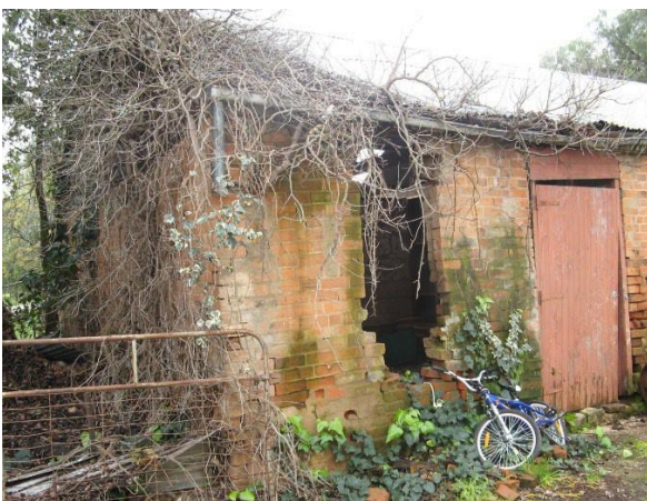
Figure 29. Plough Inn stables in 2009. (Heritage Victoria, 2009)
