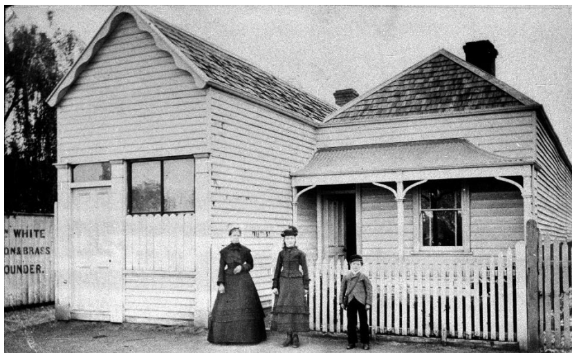
Figure 3.150 A modest foundry with attached house in Ballarat, was the premises of 'White, Iron and Brass Foundry', c.1872. (Source: State Library of New South Wales)
