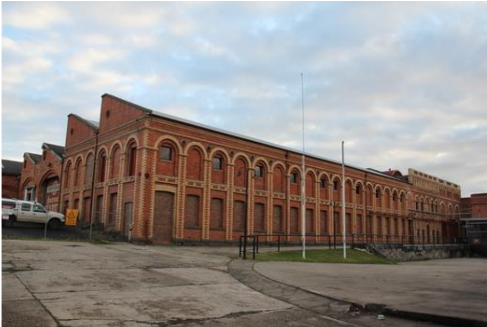
Figure 3.168 Former Sunnyside Woollen Mill, Mount Pleasant, 2011. (Source: Ballarat Heritage Services Picture Collection, photographer L.J. Gervasoni)
