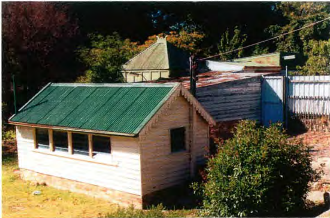
Figure 3.12 Outbuildings with the pressed metal shed at the rear.
