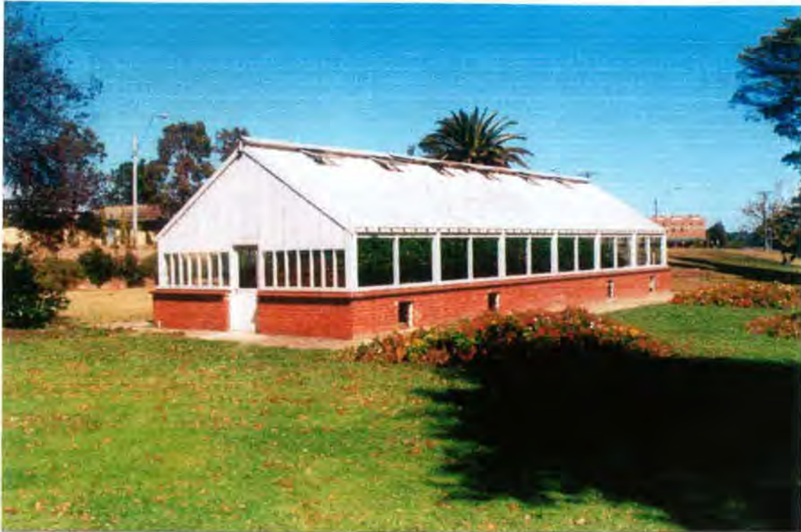
Figure 3.14 Glasshouse from north-east
