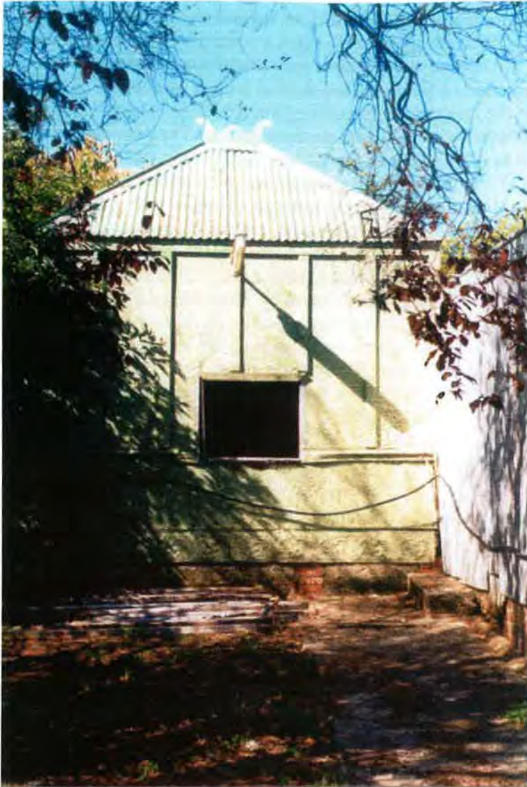
Figure 3.13 Pressed metal shed
