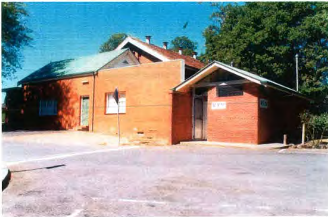
Figure 3.8 View of kitchen and toilet block from the north-west.
