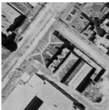
Figure 3.16 Aerial photograph from 1957 showing that the addition to the rear of the hall seen in the 1934 photograph appears to have been demolished. A detached hip-roofed building is now located to the south and an L-shaped roof form wraps from the eastern end of the hall to the south of the detached building.
