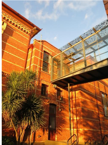
Figure 3.12 Detail, west elevation of former Free Library showing glass bridge connection to western end of the link section of the building introduced by Cox Sanderson Ness Architects as part of the 1998–2000 alterations and additions to the (then) former Ballarat Secondary College. Note that changes made to this section of the Free Library between 1957 and time of the 1998–2000 alterations and additions have sought to match the western facades of the link and hall with the original Free Library through the use of cream brick detailing to the red brick walls. (May 2020)
