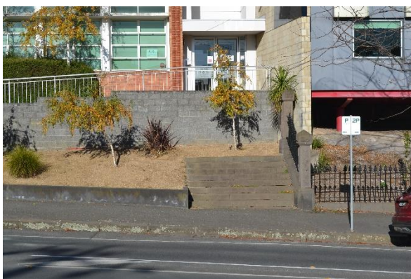
Figure 3.4 Remnant bluestone stairs in Barkly Street associated with the former Ballarat East Town Hall viewed from the north. This photograph shows the termination of these stairs by the entry ramp and landscaping introduced as part of the 1998–2000 alterations and additions to the former Ballarat Girls High School designed by Cox Sanderson Ness Architects. (May 2020)
