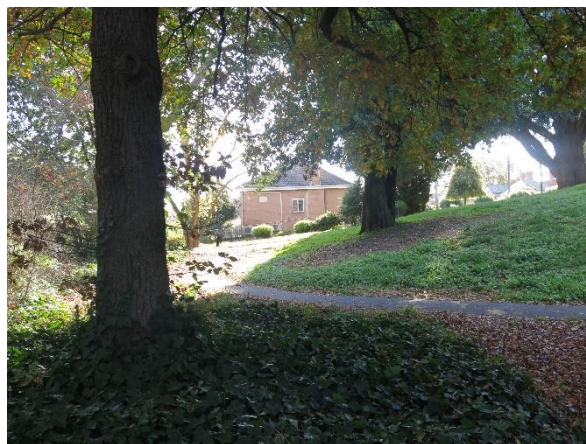
Figure 3.23 Distant view of south elevation of the former Baby Health Centre viewed from the southwest corner of the former Ballarat East Town Hall Gardens. Note single steel-framed window and chimney. (May 2020)
