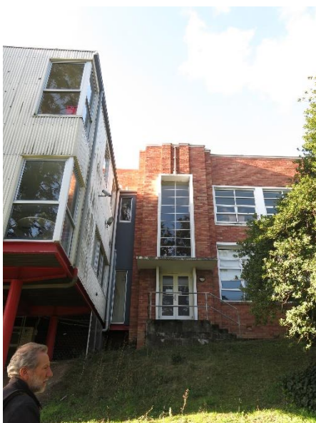
Figure 3.30 Entry, north end of west elevation of former Ballarat Girls High School. Note stepped profile, vertical composition, rectangular, flat-roofed concrete canopy and concrete landing, and steps with non-original utilitarian pipe balustrade. (May 2020)
