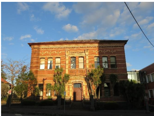
Figure 3.7 Former Ballarat East Free Library (1867–68), viewed from Barkly Street (north). The front garden contains mature cordyline and more contemporary shrubs and has an iron palisade fence set on bluestone plinths framed by bluestone piers. A central wrought iron gate arch marks the entry to the site. (May 2020)
