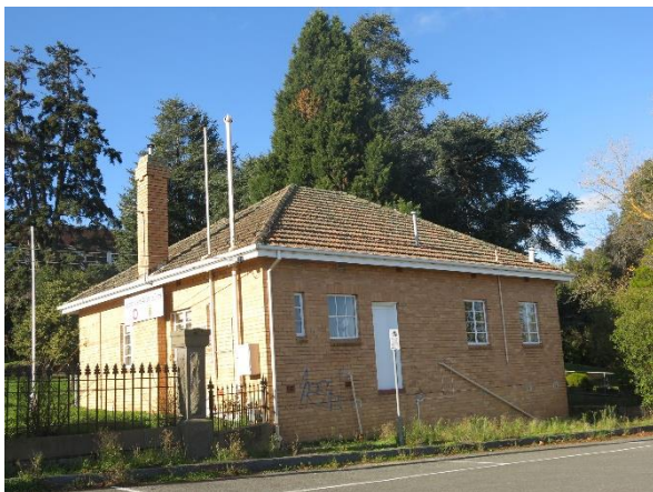
Figure 3.20 West elevation of the former Baby Health Centre. Note small steel-framed windows and rear exit door with no landing. (May 2020)
