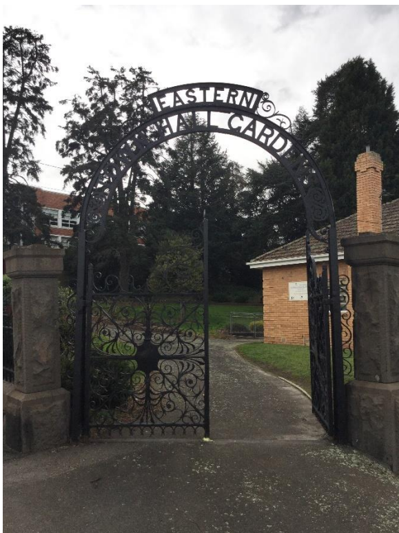
Figure 3.77 1900 entry gates to the 'Eastern Town Hall Gardens'. With no pyramidal capping evident, it is possible that the gate piers were originally intended to support lamps, such as those at the Free Library entry gates. In c.1923 the gate piers appear the same as now (see Figures 2.12 and 2.35).
