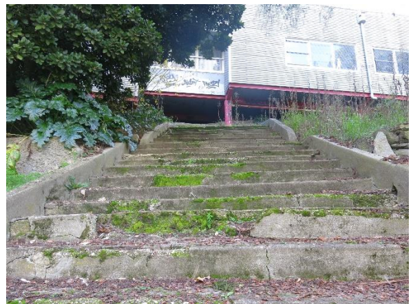
Figure 3.58 Detail of steps (2 of 3 sets). (May 2020)
