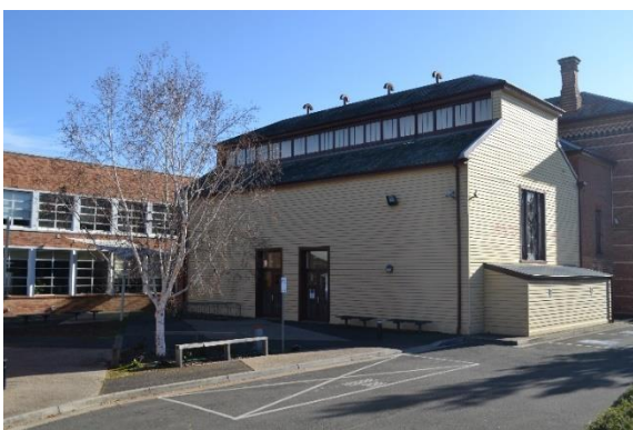
Figure 3.13 Rear (south) elevation of the rear hall showing clerestory windows, entrance doors, and weatherboard cladding to the east and south facades. A birch is located in the courtyard to the south. Eastern façade of the former Ballarat Girls High School is to the left. (June 2020)
