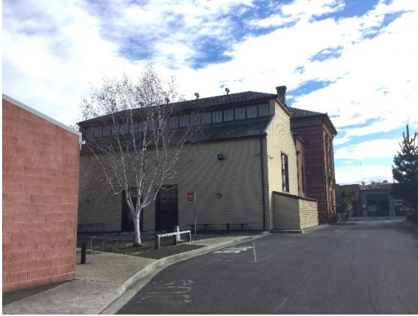
Figure 3.112 Right-of-way into the study area off Barkly Street. The right-of-way was laid out c.1857–58 (see Figure 2.6) and leads to the carpark area. It has a simple asphalt surface and concrete kerbing and guttering. Landscaping along the northern side is recent.
