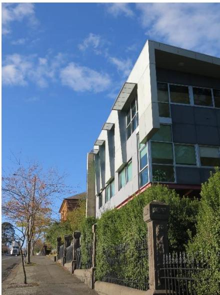
Figure 3.38 Northwest 1998–2000 extension to the Ballarat Secondary College viewed from the west. Note former Ballarat East Town Hall Garden fence in the foreground. (May 2020)
