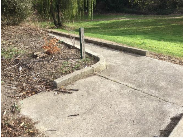
Figure 3.96 L-shaped graded pathway linking Britannia Reserve to Specimen Vale, this appears to date from the c.1950-60s and would have been associated with school use. (June 2018)
