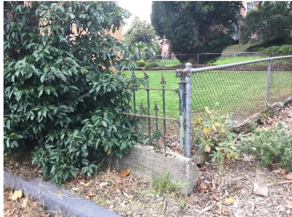
Figure 3.76 Lightweight palisade-like fencing on concrete base at rear of the Baby Health Centre and junction with steel pipe and cyclone wire fencing to the Baby Health Centre garden.
