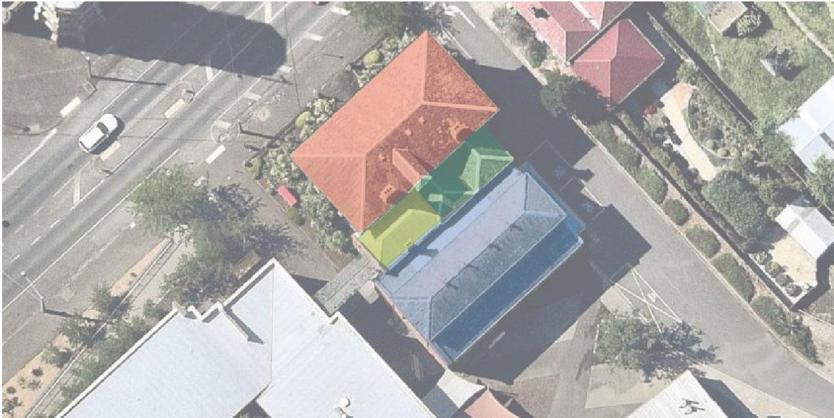
Figure 3.6 Contemporary aerial photograph of the former Free Library showing the different components of the Free Library building. The front section fronting Barkly Street (1867–68) with its east-west running hip roof and dormer to the rear is highlighted in red. The middle, or link section of the building, is highlighted in green. The eastern section of the link with its M-shaped hipped roof appears to be contemporary with the front section of the building. Evidence from historical aerial photographs of the site indicate that the western section of the link (highlighted yellow) appears to have been constructed at some time after 1957. The hall to the rear with its large hipped roof lantern is highlighted in blue. (Source: Nearmap, 2020. Annotations by Context)
