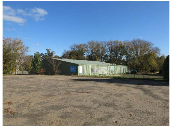
Figure 3.102 Building set back from Princes Street South frontages (built date after 1957). Set being large concrete paved area (possibly used for parking, basketball). (May 2020)
