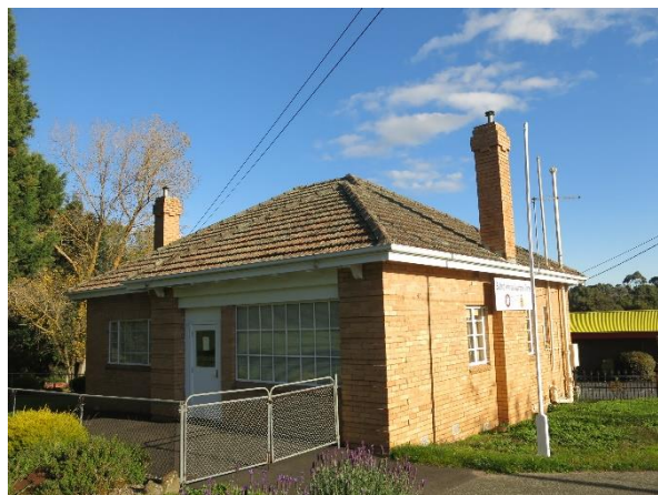
Figure 3.19 Former Baby Health Centre, showing the projecting bay to the north end of its east elevation. Note the distinctive brick banding, entrance door, multipaned steel windows with brick sills and chimneys with stepped capping.
