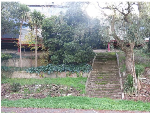
Figure 3.57 Terracing with stone and rough rendered retaining walls, and steps (2 of 3 sets). Stairs no longer provide access to school building. (May 2020)
