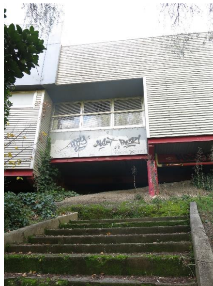
Figure 3.41 Detail of the southern elevation of 1998–2000 extensions to the Ballarat Secondary College. Concrete stairs associated with former Ballarat Girls High School era in the foreground. (May 2020)
