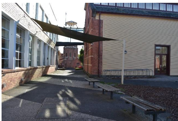
Figure 3.14 View of the Free Library and rear hall (right) and former Ballarat Girls High School (left) from the south. Note timber weatherboard cladding to south elevation of hall and banded brick elevation to west. Ballarat East Fire Station can be seen in the background. (June 2020)
