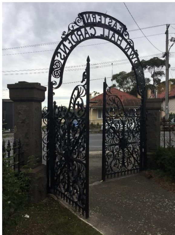
Figure 3.78 Reverse side of entry gates from inside the garden.
