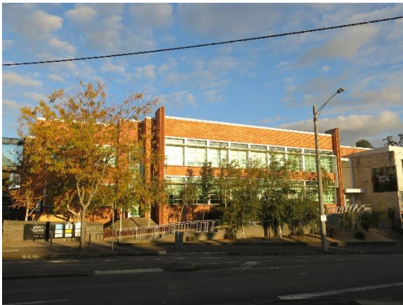
Figure 3.26 1955 former Ballarat Girls High School building. Note ramp to entrance between the 1955 School and the 2000 additions carried out to the (then) Ballarat Secondary College (right) in 2000. The line of birches and landscaping appear to be recent additions associated with the 2000 works. (July 2019)
