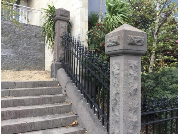
Figure 3.63 Remaining section of early palisade fence on bluestone base with bluestone piers with rusticated panels (section on opposite of the steps is no longer extant).
