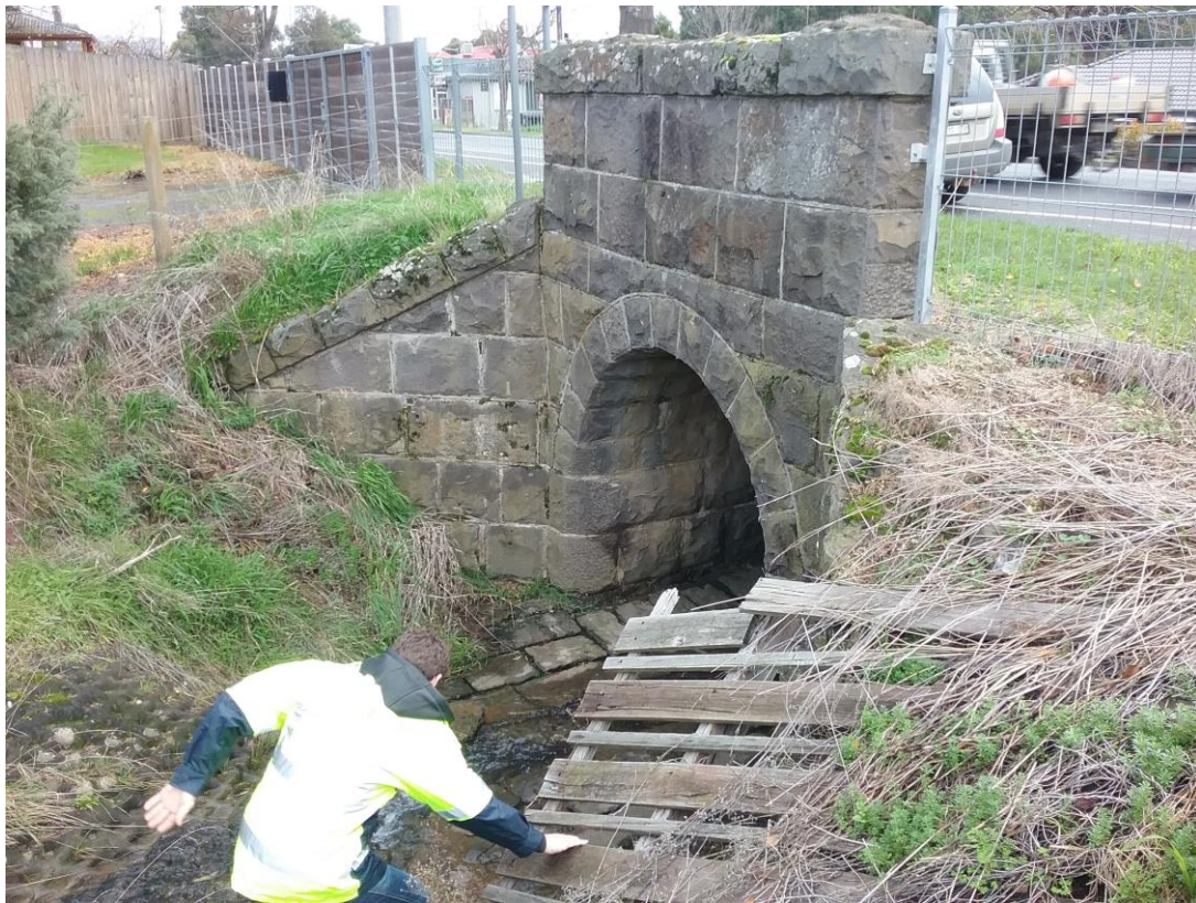
FIGURE 2-2 HUMFFRAY STREET NORTH CULVERT ON WARRENHEIP CREEK (DOWNSTREAM)
