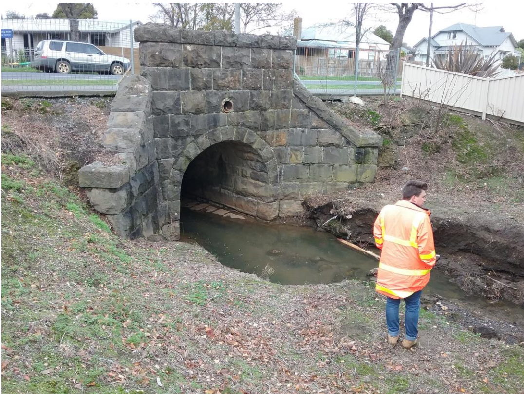
FIGURE 2-1 HUMFFRAY STREET NORTH CULVERT ON WARRENHEIP CREEK (UPSTREAM)
