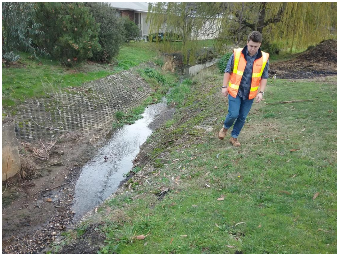
FIGURE 2-3 WATER STREET CULVERT ON WARRENHEIP CREEK (DOWNSTREAM)
