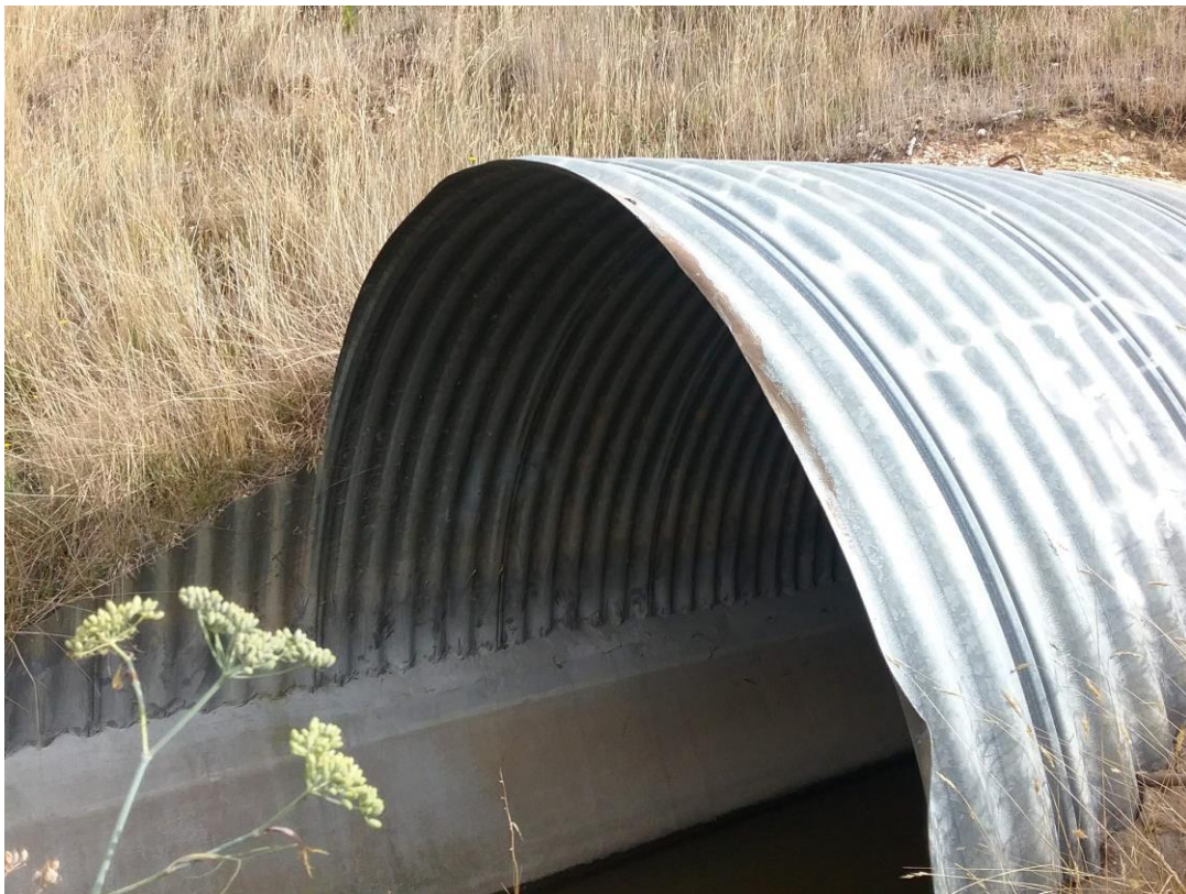
Figure 4-6 Culvert Pit located at “A” (top); Large Culvert Located at “B” (bottom)
