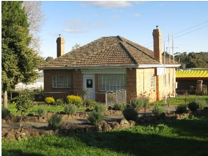
Figure 3.258 Ballarat East Infant Welfare Centre, designed by the Public Works Department architect Percy Everett, was opened in 1938. (Source: Context, 2020)
