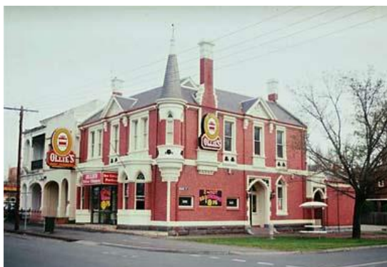
Figure 3.248 Former doctor's residence, 802 Sturt Street, Ballarat Central. (VHD?)
