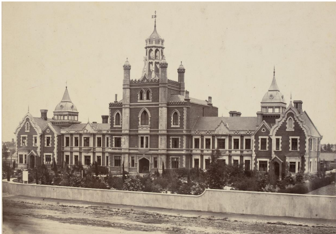
Figure 3.250 Ballarat Benevolent Asylum, built in Ascot Street, Ballarat West, in the 1850s. (Source: State Library Victoria, Accession No. H1786)
