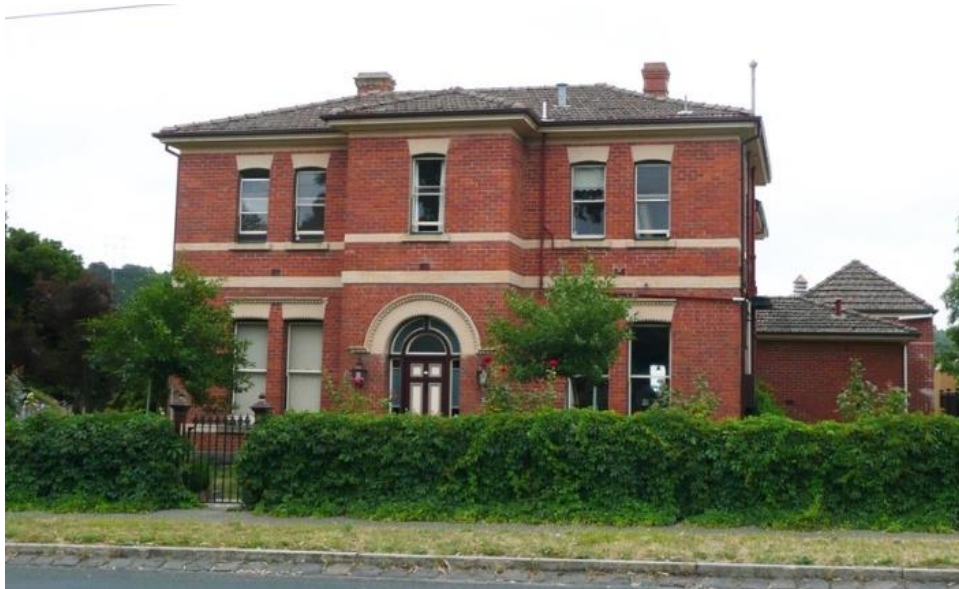
Figure 3.251 Former Female Refuge, 183 Scott Street, Ballarat East; photographed in 2008. (Source: Victorian Heritage Database)
