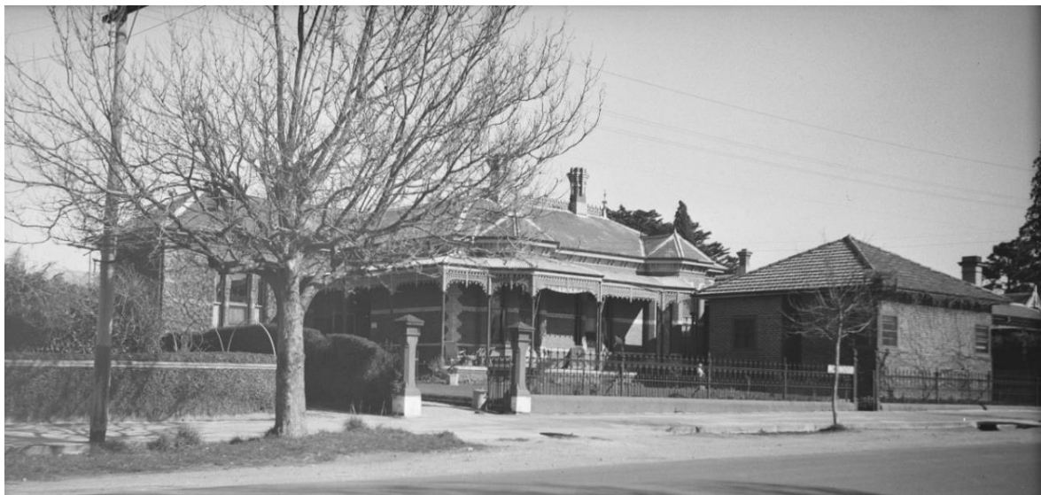
Figure 3.247 Norwood private hospital, Ballarat. (Source: PROV)
