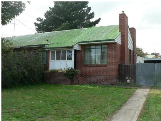
Figure 3.254 Brick veneer Housing Commission house in Hurley Street, Ballarat North. (Source: Realestate.com)
