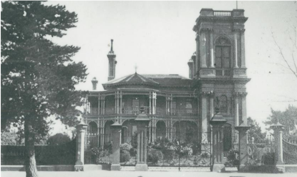
Figure 3.244 The former mansion of William Bailey at Lake Wendouree was acquired for the establishment of the St John of God Hospital. (Source: St John of God Ballarat website)
