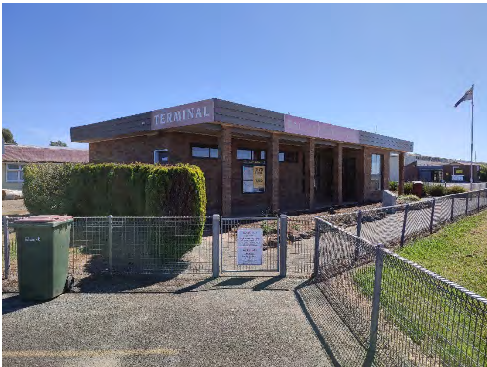
Figure 38: Existing Terminal Building
