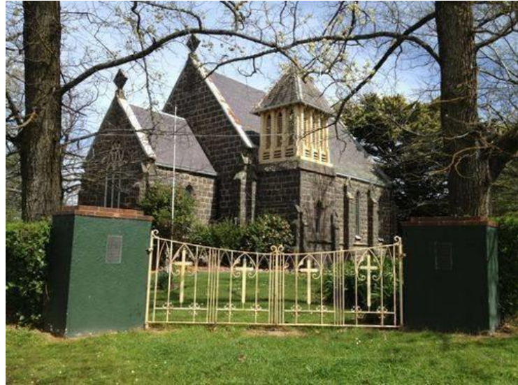
Figure 3.175 Holy Trinity Anglican Church, Buninyong. (Source: Monument Australia)
