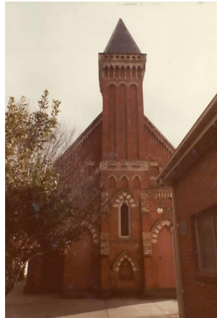
Figure 3.194 St John's Lutheran Church, Doveton Street South, Ballarat. (Source: National Trust of Australia (Vic), B4717)
