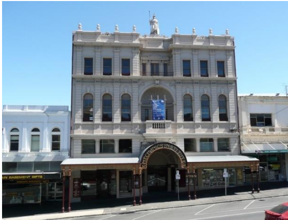
Figure 3.203 Ballarat Mechanics Institute, Sturt Street, built in 1859. (Source: VHD)
