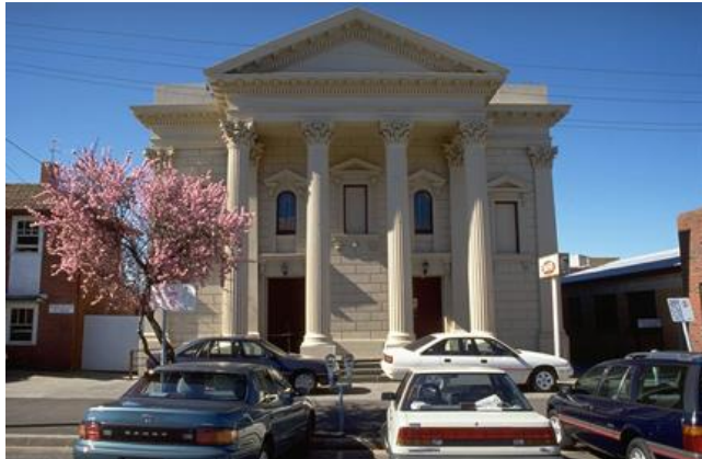
Figure 3.192 The imposing Classical Revival design of the Baptist Church, Ballarat Central, built c.1866–67; the front section was added later. (Source: RNE)
