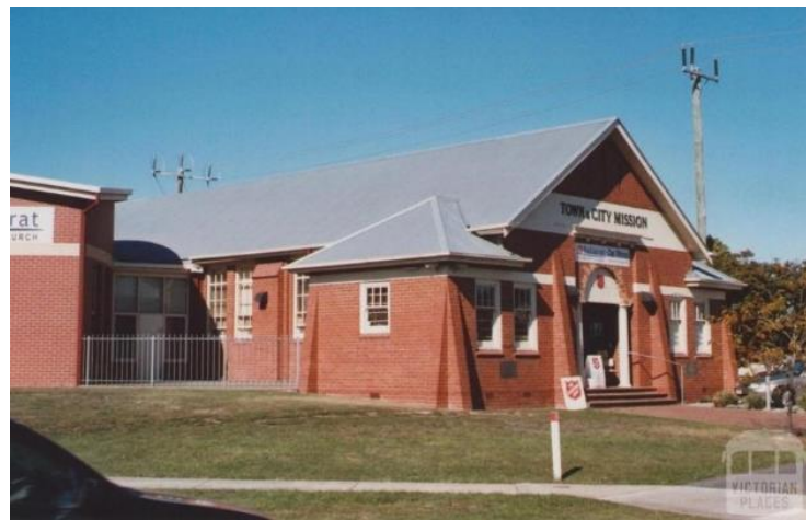
Figure 3.196 Salvation Army Mission building, Ballarat East, built c.1916–20. (Source: Victorian Places, 'Ballarat East')
