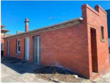
Laundry viewed from the southwest
