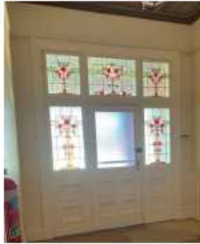
Front entrance of the house viewed from the front hall
